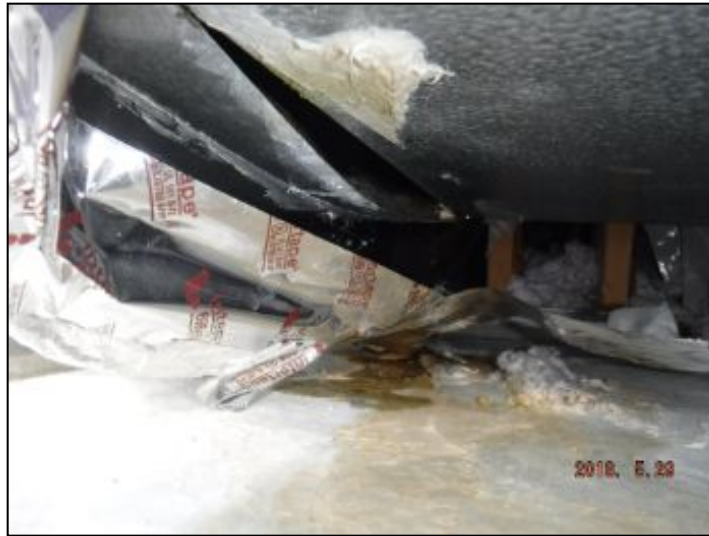
leaking plenum
