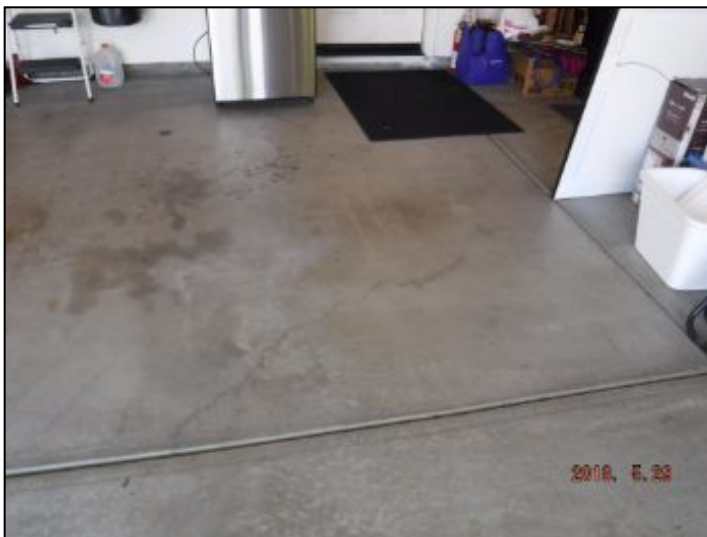
typical cracks
