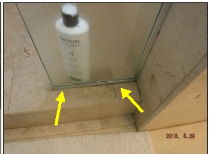
leaking enclosure
