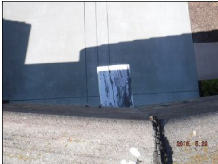
exposed beams (ok)
