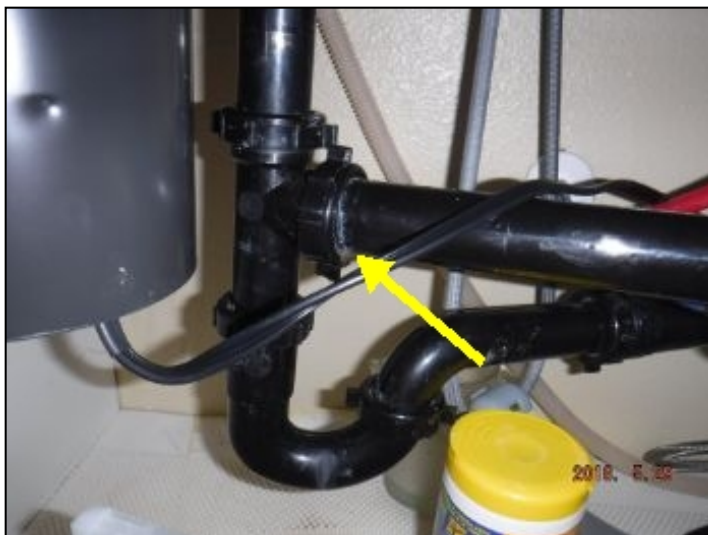
drain leak
