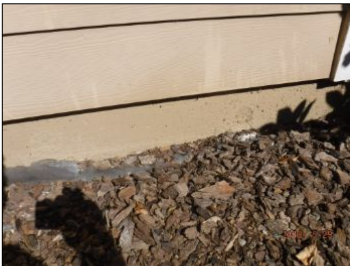
post tension slab foundation
