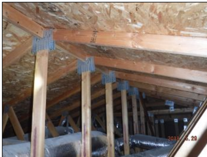
attic framing ok
