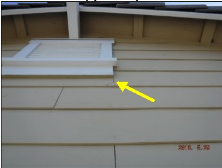
cracked siding
