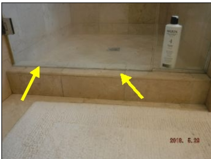
missing wiper seal
